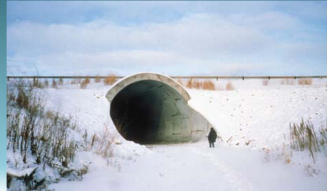
Inlet of new culvert, following winter.
